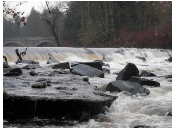
Lower flow conditions on 21 January 2016 River level 0.67 m, flow 7.63 m 3 /s, Q20 approx.
