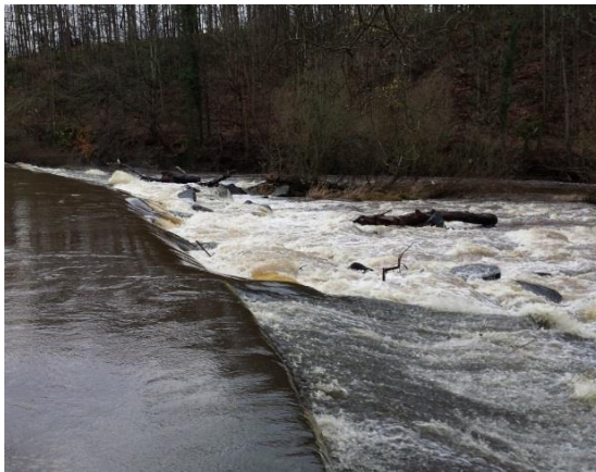
High flow conditions on 11 December 2015 River level 1.2 m, Flow 22.5 m 3 /s, Q5 approx.
