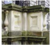
Where indenting is appropriate, the indent should be selected to closely match the original stone. Artificial stone should not be used on listed buildings.
