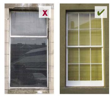
Care should be taken the ensure that replacement windows are fitted in the same plane as the originals, are made of timber sections (the profile and dimensions of which match the originals) and have the meeting rails in the same position as the originals; this is especially important where the windows of only one property in a tenement or terrace block are being replaced.
