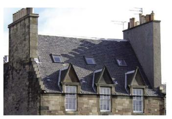
The roof, which includes parapets, skews, chimney heads and chimney pots, is an important feature of a building. The retention of original structure, shape, pitch, cladding (particularly colour, weight, texture and origin of slate and ridge material) and ornament is important. Any later work of definite quality which makes a positive contribution to the interest of the building should also be kept. The restoration of lost roof elements to match the original form will be encouraged.
