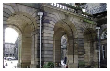
Replacement rainwater goods should match the original, cast iron or zinc should be used where these were the original materials. Other materials such as aluminium may be acceptable, where appropriate.
