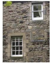
glazing bar with flush flashings preferably top hung. Alternative materials such as uPVC will not be acceptable.
