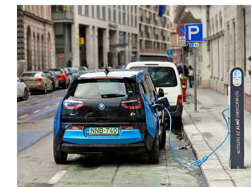
Electric car charging points
