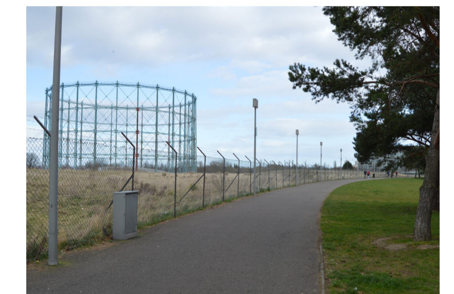
Existing disconnection to the waterfront
