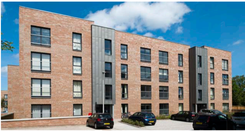
Former Niddrie Mill Primary School
