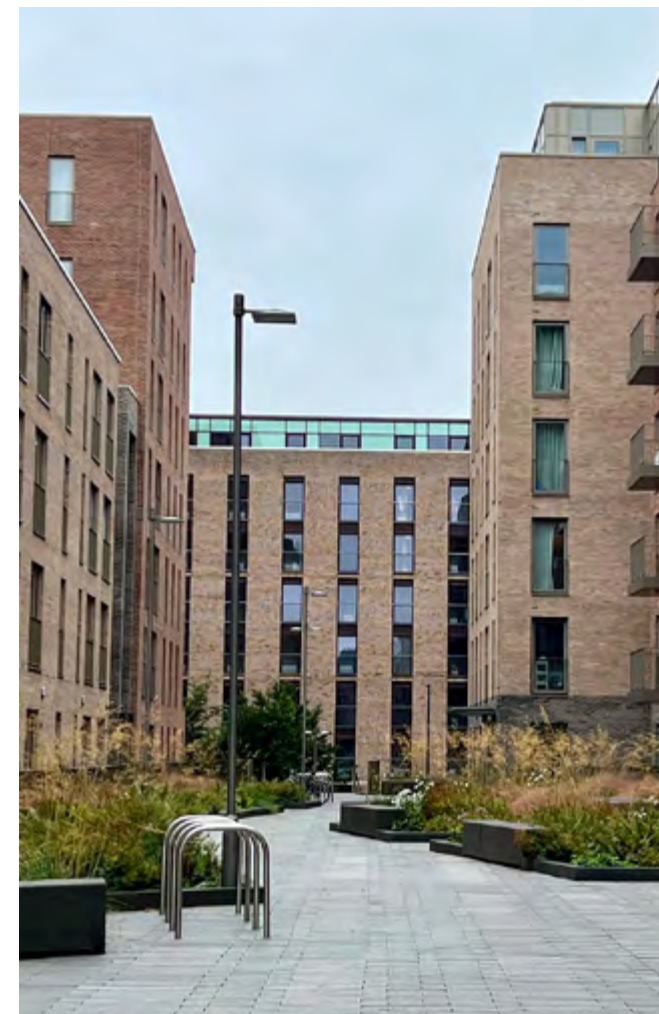
Nature-based solutions: Rain Gardens - McEwan Walk in Fountainbridge uses rain gardens to manage rainwater and address the risk of flooding. They also enhance the overall quality of the public realm.
