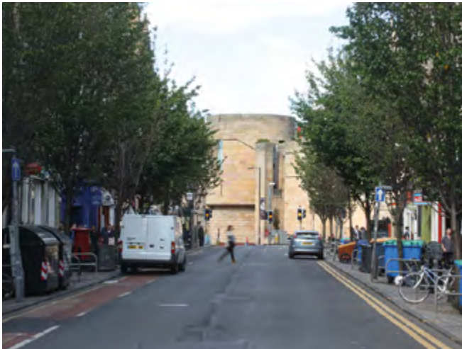
Forrest Road: This street extends the tree lined avenue of Middle Meadow Walk to George IV Bridge
