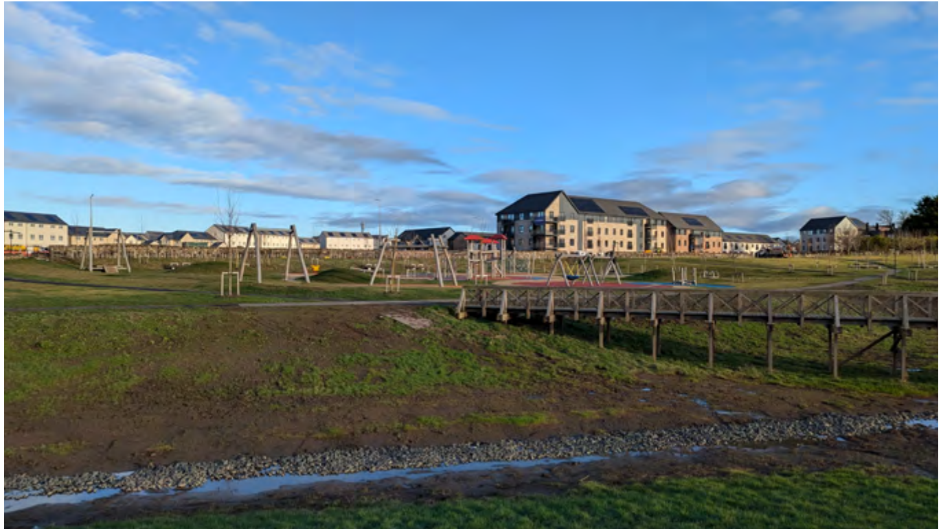
SuDS integrated from the outset - Sustainable rainwater management was considered from early in the design process of Meadowfield Park in West Craigs. It forms an integral part of the wider park. The park has been designed with a raised timber walkway and wildflower meadow planting.
