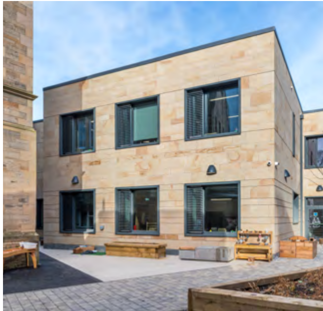
Minimising embodied energy of new buildings - The extension to Sciennes Primary School was constructed using stone-clad exposed cross-laminate timber (CLT). The use of CLT minimised the embodied energy by using natural materials that contribute to carbon storage. By exposing the CLT internally a comfortable environment was created without needing additional internal finishing. The extension was also designed to Passivhaus standard, reducing the operational energy consumption of the scheme. The external stone cladding responded to the setting of the extension next to a category B listed building in the Marchmont Conservation Area. Photos courtesy of Holmes Miller, © Chris Humphreys Photography.
