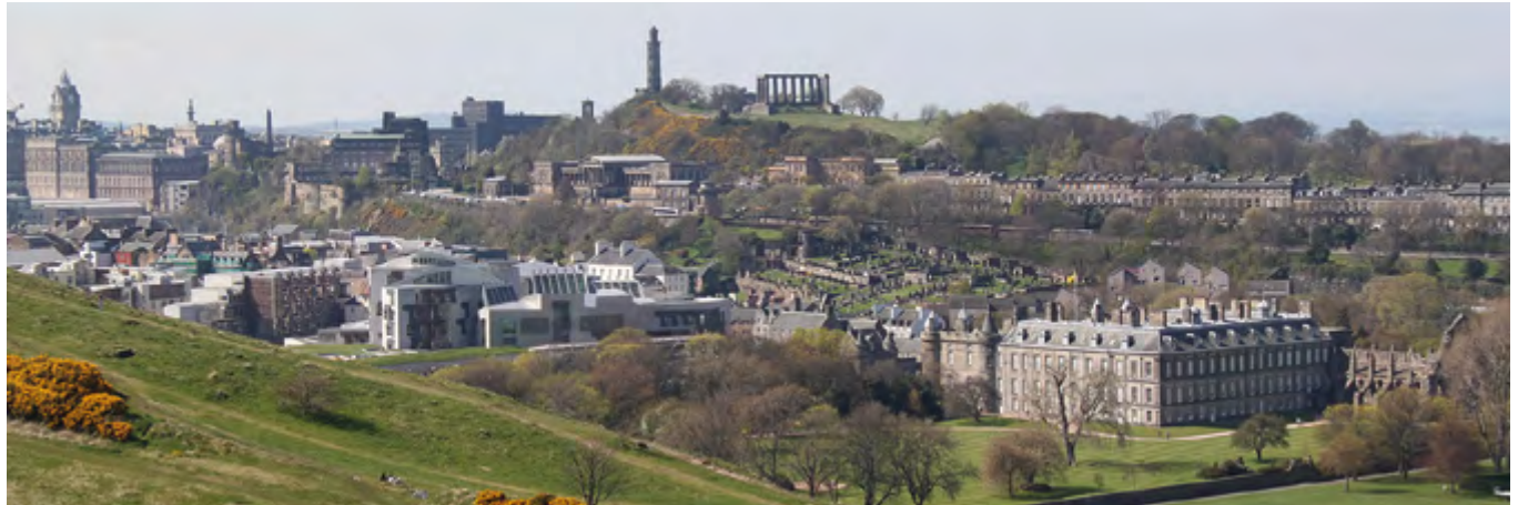
Protecting Edinburgh's Skyline - The view of Calton Hill from west escarpment of Long Row, Whinny Hill is protected (view no. E05)
