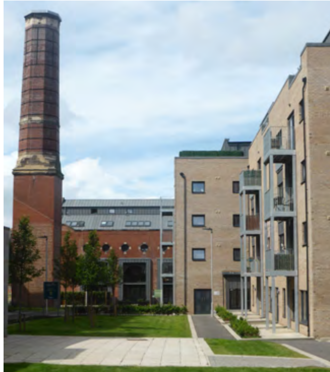
Retention of existing buildings - As part of the redevelopment of the former engine yards at Shrubhill, the conversion of the redundant tram sheds has safeguarded an important landmark that makes a special contribution to the surrounding area, while retaining the embodied carbon of the buildings.
