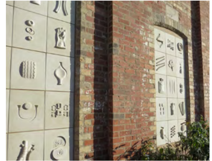
Artwork referring to a building's history - The cast concrete artwork 'Catalogue Wall' by Mark Doyle is located on the wall of Edinburgh Printmakers. It references the history of this former rubber factory and the products it manufactured.
