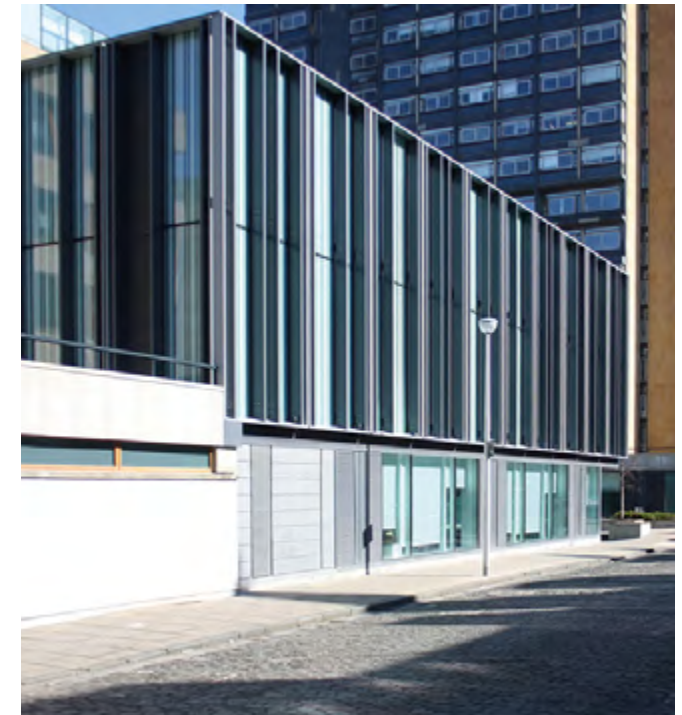
Curtain Walling: Buccleuch Place - The potential offered by glazing systems with variations in the window widths, patterning of the glass and mullion depths is fully taken advantage of here.
