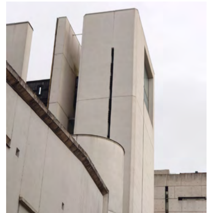
Sculptural concrete - In-situ concrete is used on the Museum of Scotland building to create a sculptural effect.
