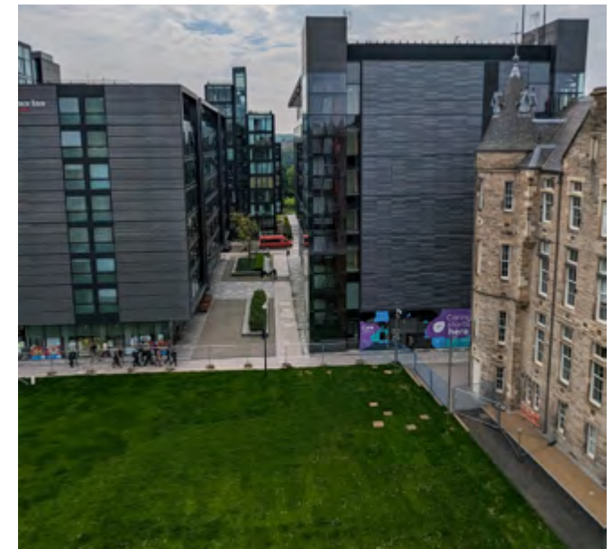
High-density supporting a mix of uses - the density of the development at Quartermile supports a range of ground floor uses.
