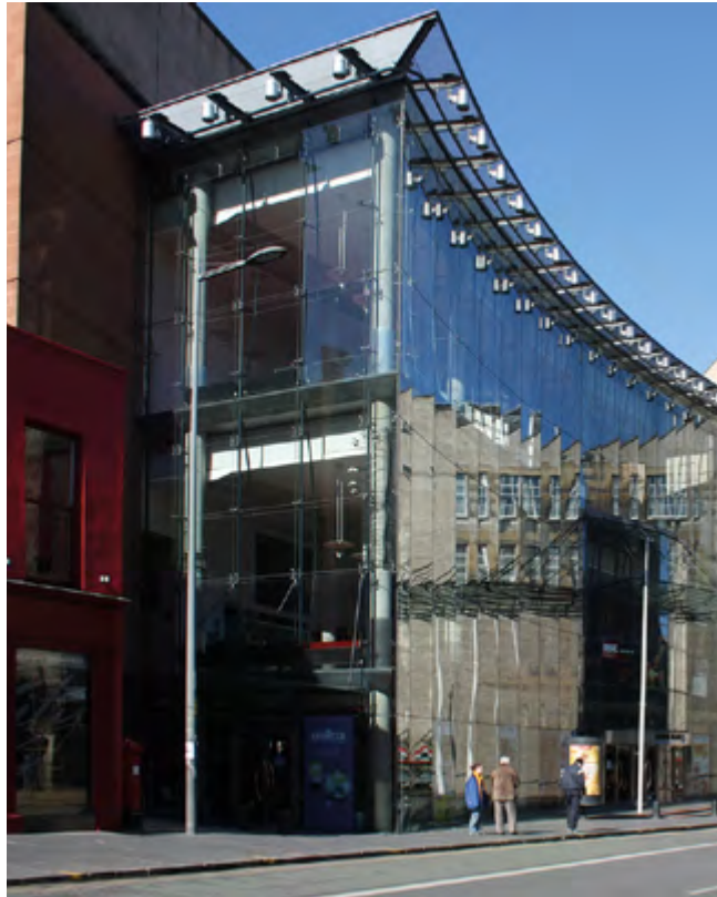
Frameless glazing: Festival Theatre, Nicolson Street - The refined detailing of the frameless glazing helps create a striking modern addition to the street.
