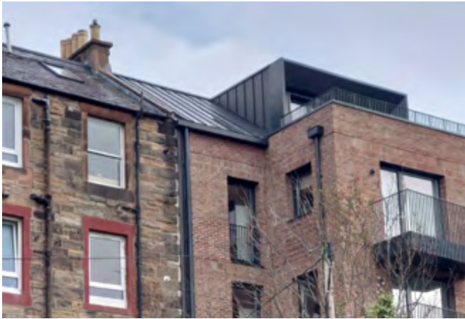
Taking cues from neighbouring heights - The height and roof pitch of this new building is designed to match the height and roof pitch of the adjacent building.
