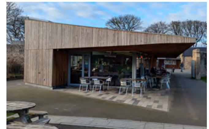
Creative timber cladding - This new timber-clad garden café at Saughton Park forms part of the conversion of the stable block into a popular community hub.
