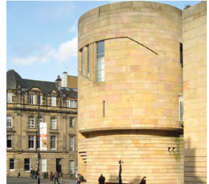
Sculptural and contextual stone cladding - At the Museum of Scotland rigorous and sculptural use of sandstone cladding provides the building with a striking contemporary aesthetic that responds positively to the surrounding historic context. Care needs to be taken with any proposal like this, that the detailing mitigates adverse weathering and staining.
