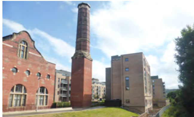
High-density responding to historic context - The density of Shrubhill responds well to the heritage and character of the area.
