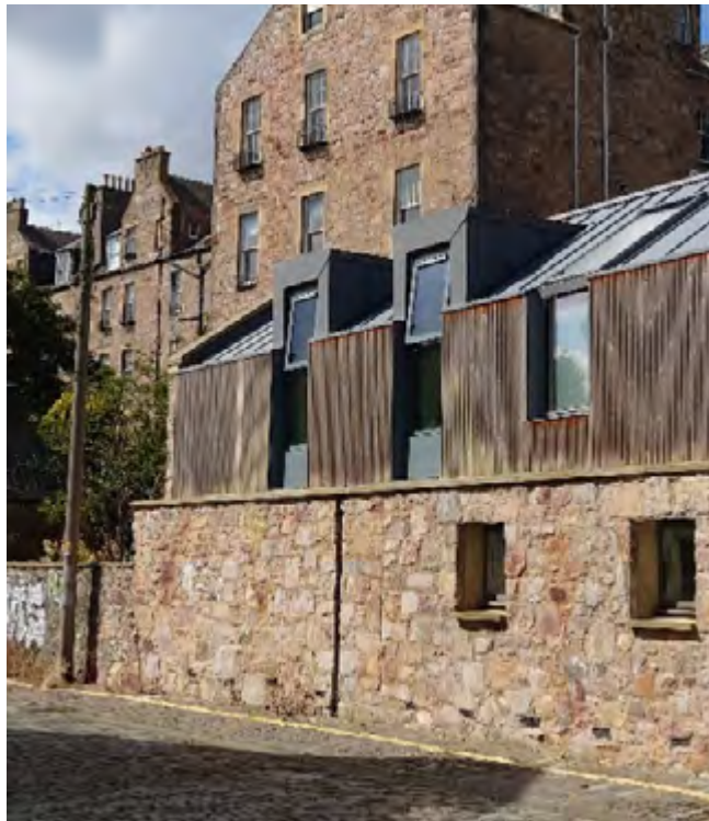
Timber and stone: Meadow Lane - Timber cladding to the upper floor of this mews development provides a positive contrast to the stone base that adds visual interest to the lane.
