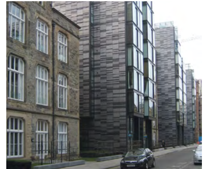
Aluminium: Simpson Loan - Multi-toned anodised aluminium cladding provides a striking and positive contrast to the historic buildings making the distinction between new and old very clear.
