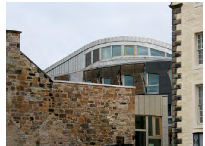
Metal roofing in a historic context: Canongate - Stainless Steel roofing has been used on the Scottish Parliament.
