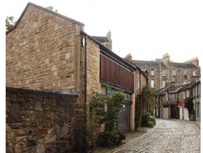
Matching the height of existing mews: Circus Lane - This newly built house matches the eaves and ridge heights of the adjacent historic mews buildings.
