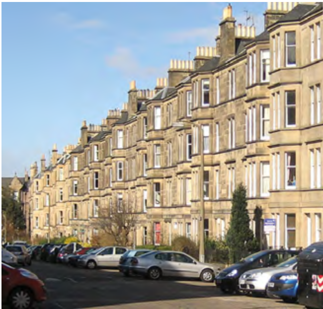
Generous window heights: Marchmont, Arden Street - These tenements manage to provide good levels of daylight to all the properties. This is a result of the high floor to ceiling heights and relatively large and tall windows which allow daylight to go deep into the rooms.
