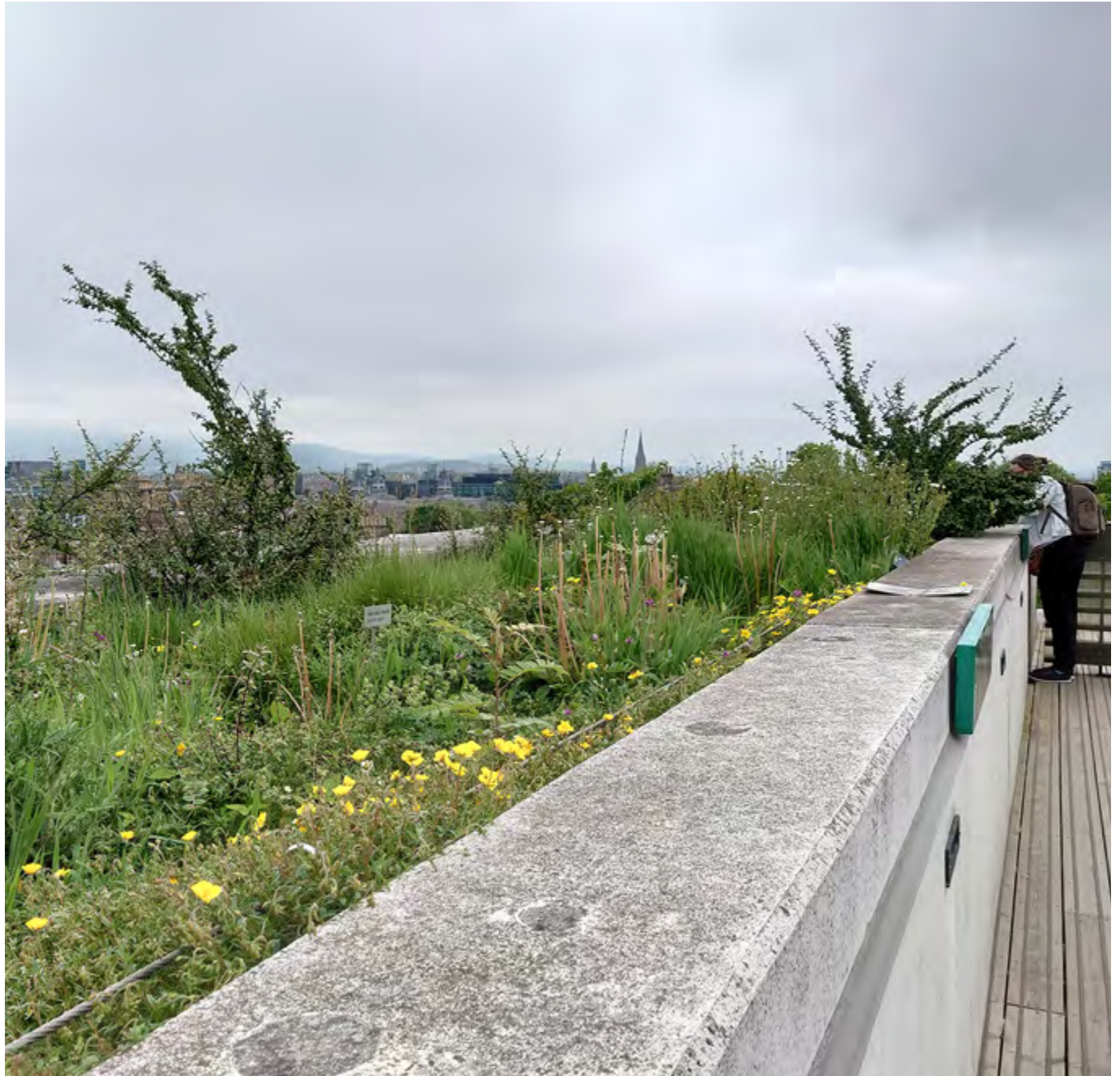
Rooftop planting to reduce risk - The intensive planting on the rooftop of the National Museum of Scotland provides an attractive edge, while also delaying or deterring anyone from accessing the roof edge.
