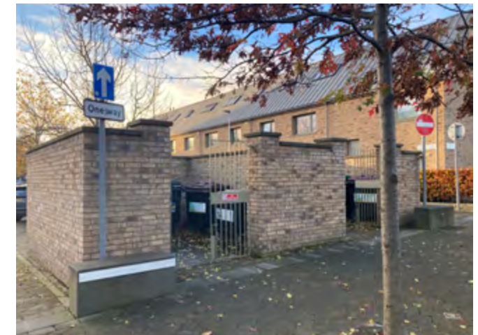
Accessible bin enclosures, Leith Fort - These carefully designed bin stores are discrete but easily accessible
