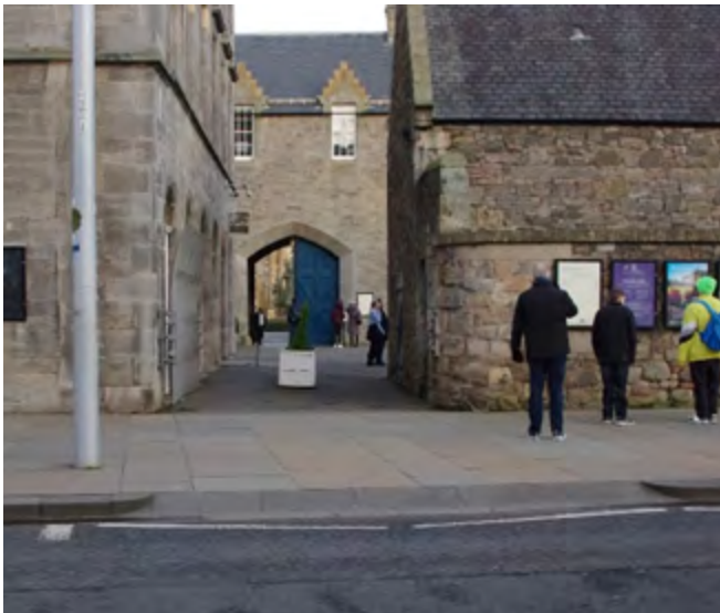
Vehicle crossovers on footways - This vehicle crossover on Horse Wynd maintains a level footway suitable for wheeling. Vehicle crossovers (e.g. to access driveways) that slope the entire footway down can make journeys with a wheelchair or buggy difficult.
