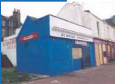
Vacant Commercial premises at the Promenade
