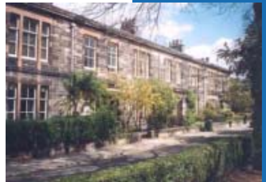
Mid 19th Century properties on Elcho Terrace
