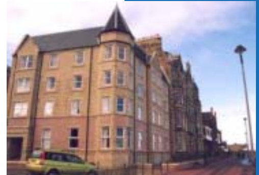
New development on Pitville Street/Promenade
