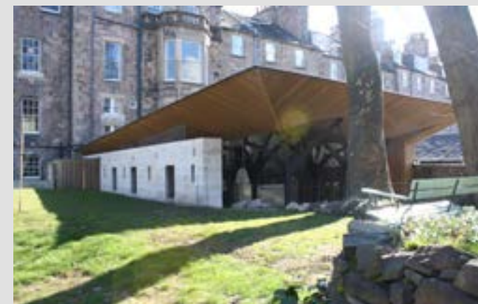
Frameless glazing—George Square Lane Glazing is used to create the effect of a floating roof on this religious building
