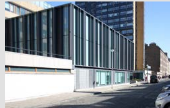
Curtain Walling—Beccleuch Place The potential offered by glazing systems with variations in the window widths, patterning of the glass and mullion depths is fully taken advantage of here.
