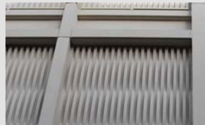
Textures created with concrete—Princes Street Concrete panels with textured surface treatment are used on this recent building on Princes Street.
